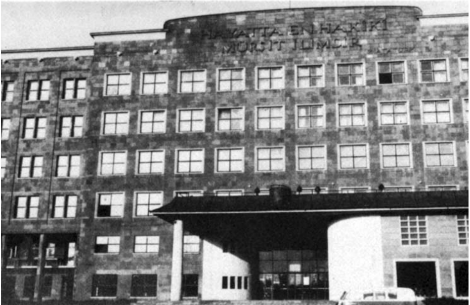
Fig. 7 New education buildings of Ankara. Ismet Pařa Girls' Institute (above); Faculty of Humanities (below). Source: Sözen-Tapan, 1973.
