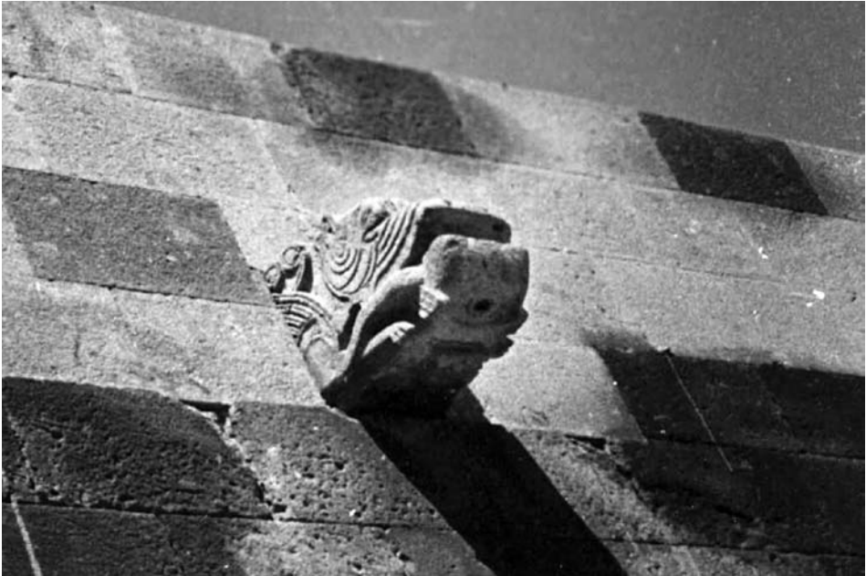
Fig. 5 Water spout from Karatay Han near Kayseri. Source: M. Önge photo archive.
