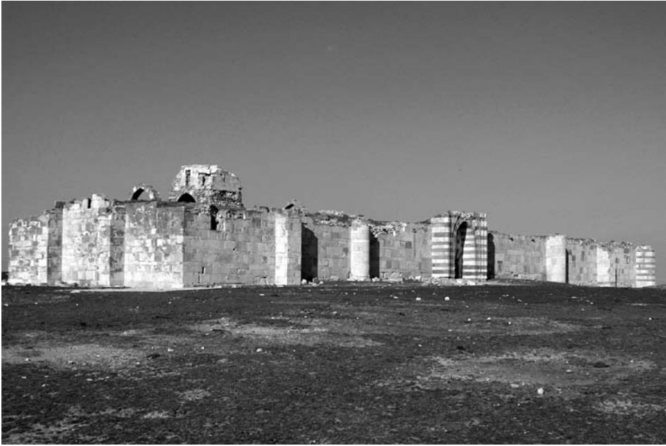
Fig. 4 Sadeddin Han, South and west facades. Source: M. Önge photo archive.
