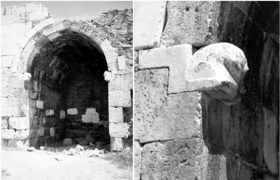
Fig. 7 Springers at the iwan of Ak Han near Denizli. Source: M. Önge photo archive.
